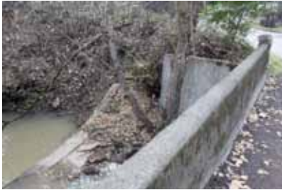
Bridge over Stevens Creek
