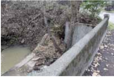
Bridge over Stevens Creek
