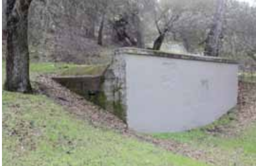
Historic water tank
