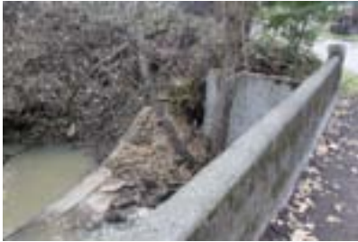
Bridge over Stevens Creek
